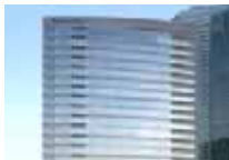
Heating & Ventilation A/C Company Headquarters
